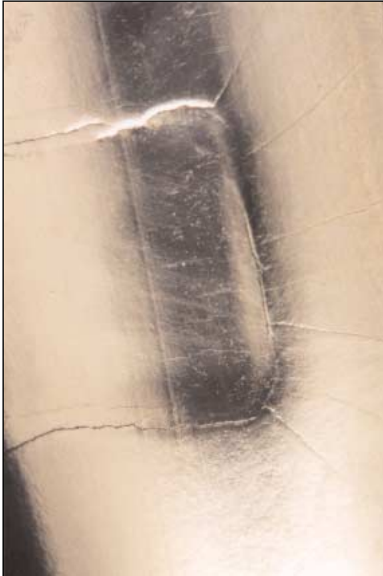
CLAMP INDUCED CRACKS IN SURFACE OVERLAY OF A "SPRAY METAL" POLISHED ROD
